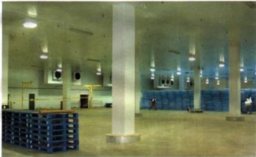
Dairy Crest's new site is cooled by a secondary system employing Tyfoxit secondary coolant
