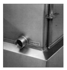
**Overflow Connection** Each chiller has an overflow connection to guard against over-filling the reservoir.
